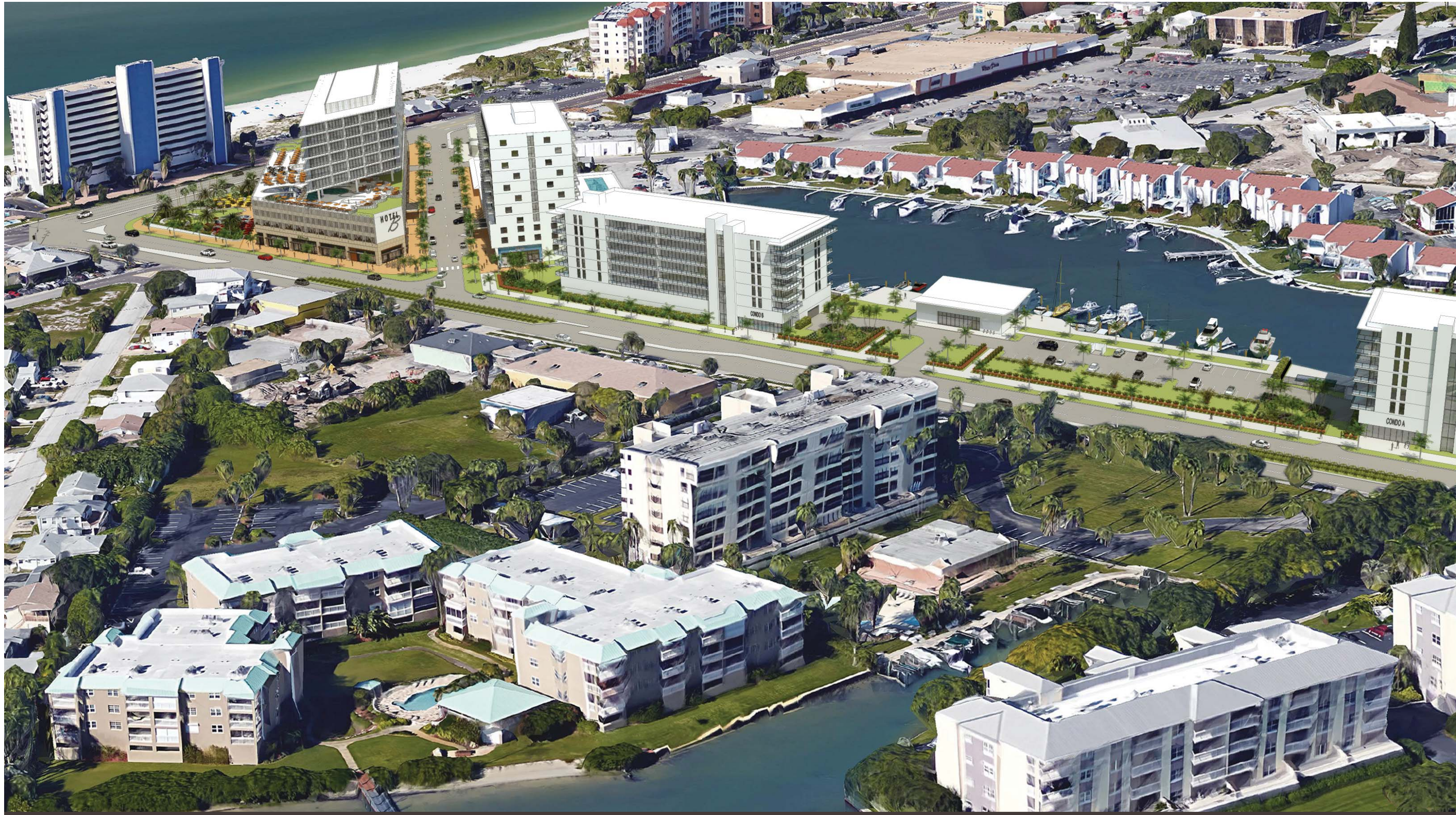
AERIAL VIEW FROM EAST
